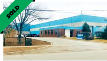
326 Clarence Road, BRAMPTON
